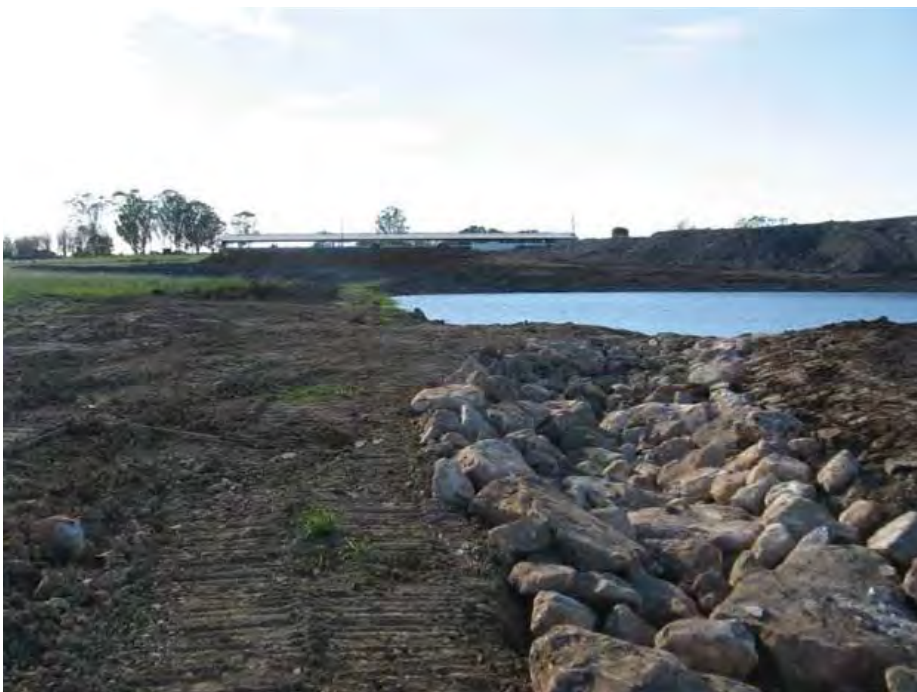
Sedimentation Pond 4 after being de-silted and refurbished
