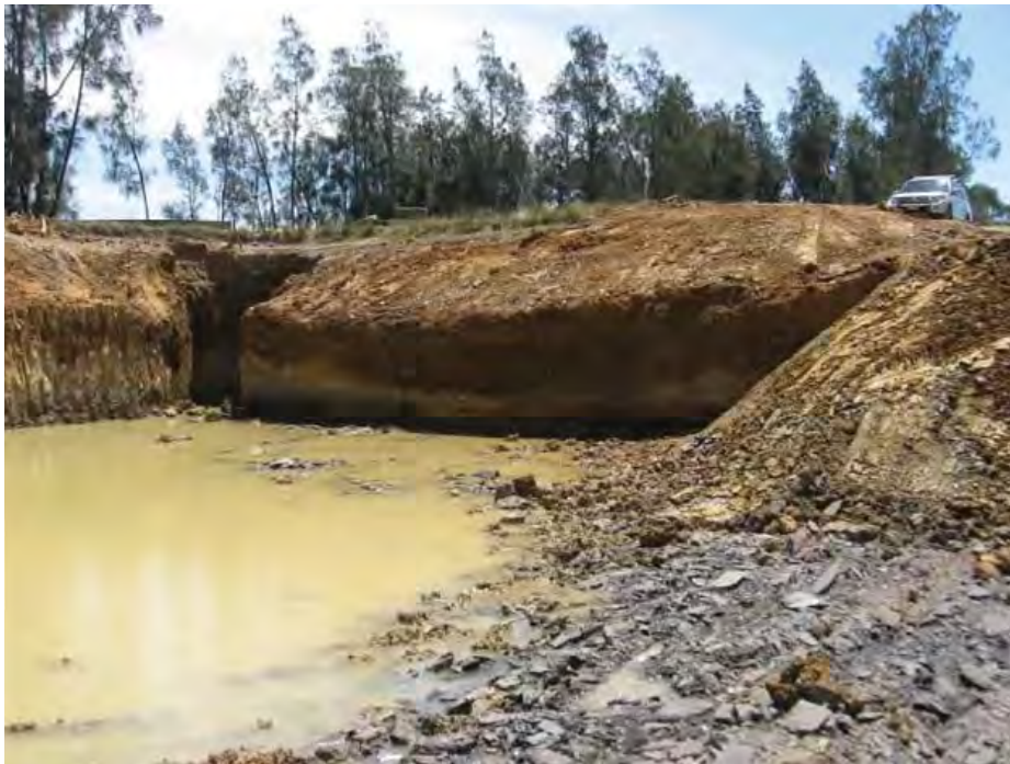
Sedimentation Pond 3 being de-silted
