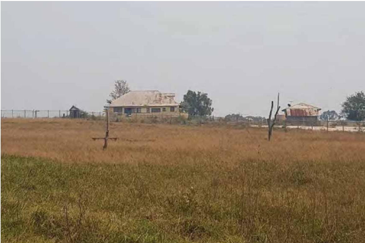
Photograph 6.2 View from northern portion of site to offsite condemned uninhabited residence (on left) and smaller unoccupied residence on right
