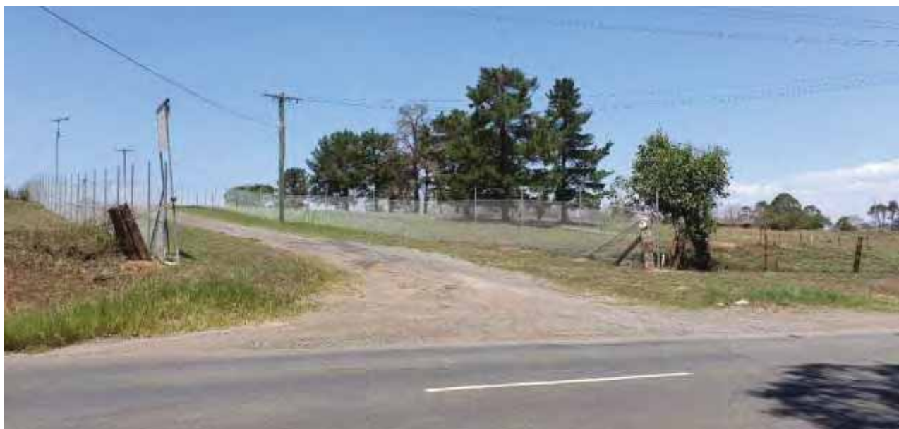
Photograph 6.1 Existing driveway off Adams Road
