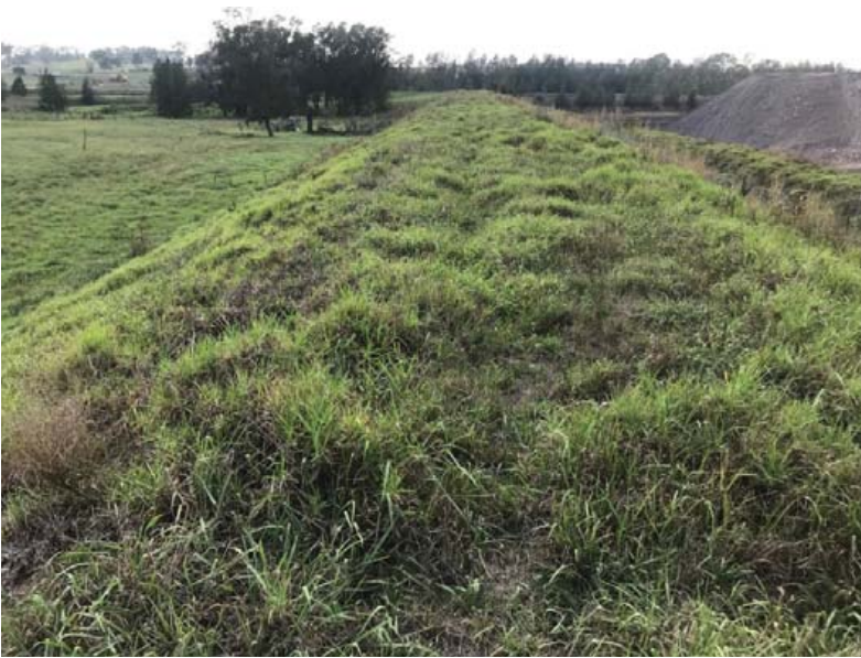
Photograph 2.1 Northern noise bund
