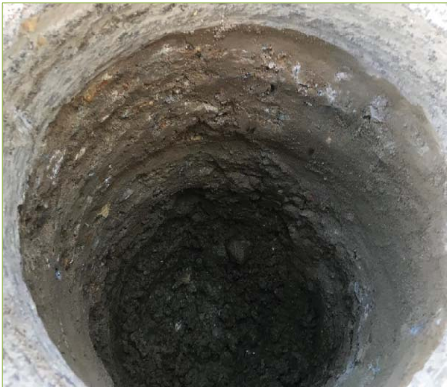
Figure 2.2.2 – BH1: Existing Pavement Structure
