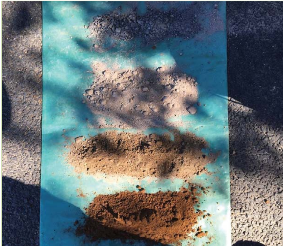
Figure 2.2.15 – BH5: Existing Pavement Materials (Top to Bottom)
