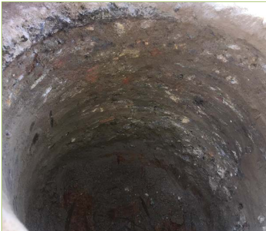
Figure 2.2.8 – BH3: Existing Pavement Structure
