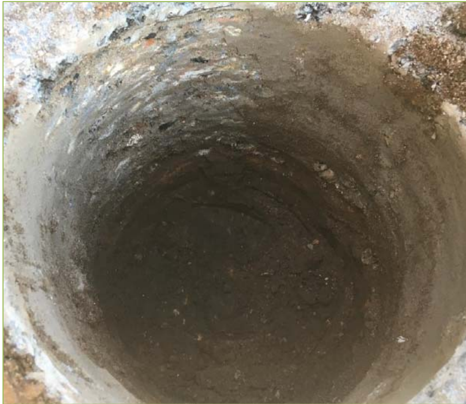
Figure 2.2.5 – BH2: Existing Pavement Structure
