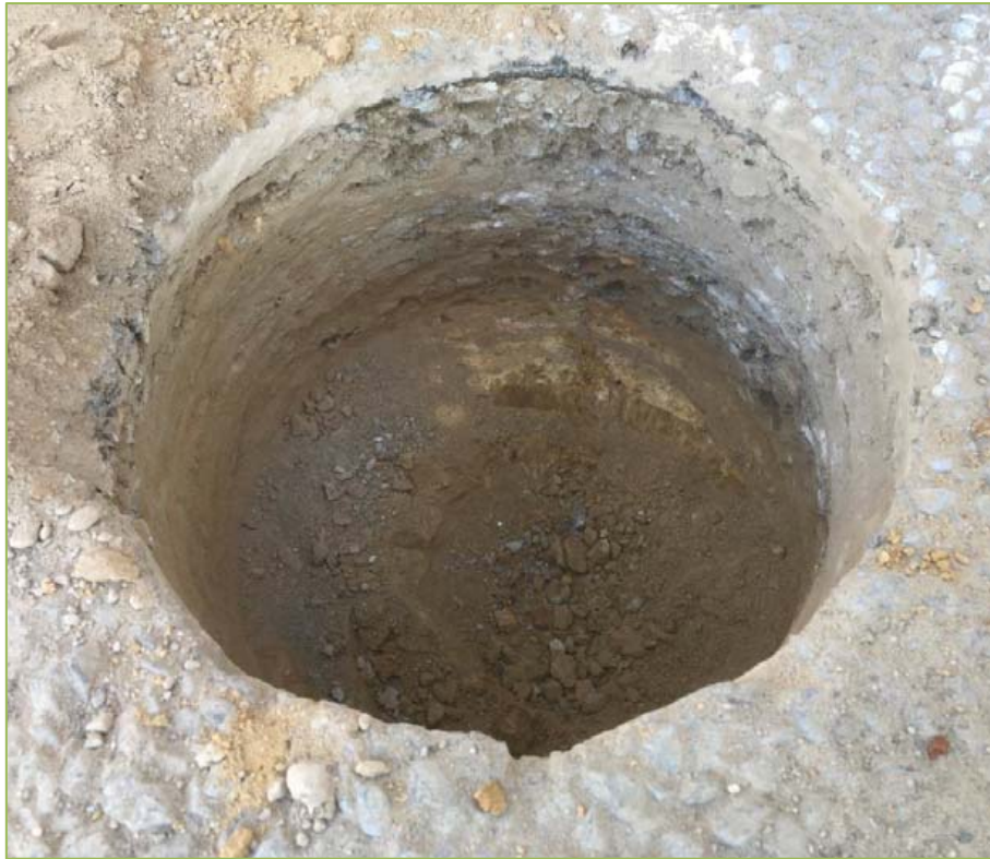
Figure 2.2.11 – BH4: Existing Pavement Structure
