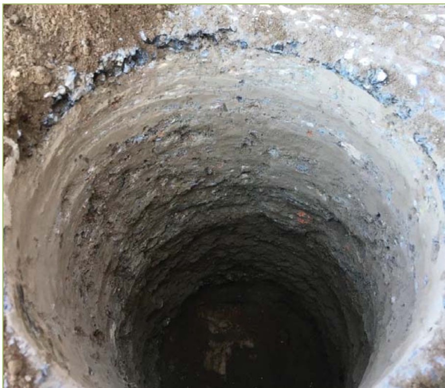
Figure 2.2.14 – BH5: Existing Pavement Structure
