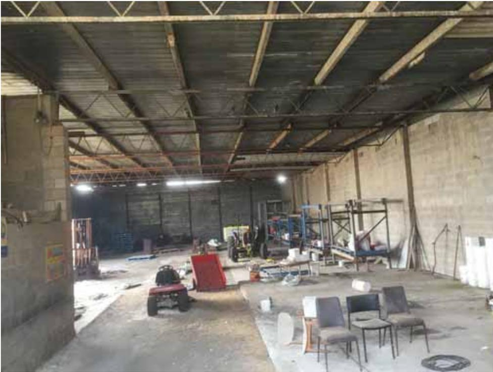
**Photograph 5.7** Inside of disused farm shed showing metal truss and roofing
