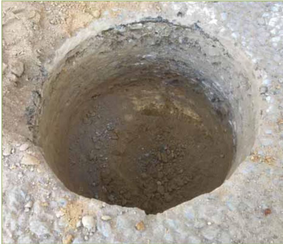
Figure 2.2.11 – BH4: Existing Pavement Structure
