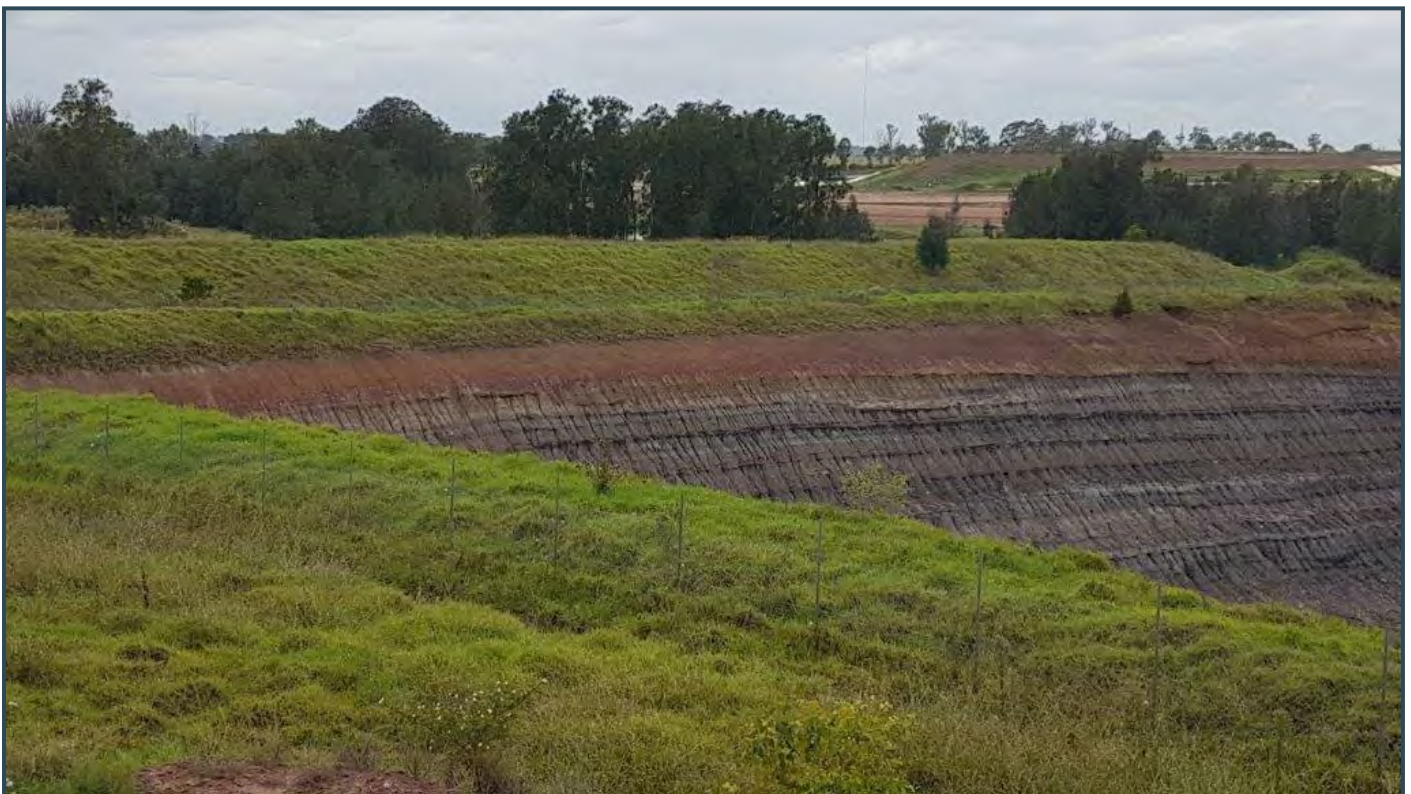
Photoplate 4. Northern Bundwall Stabilisation
