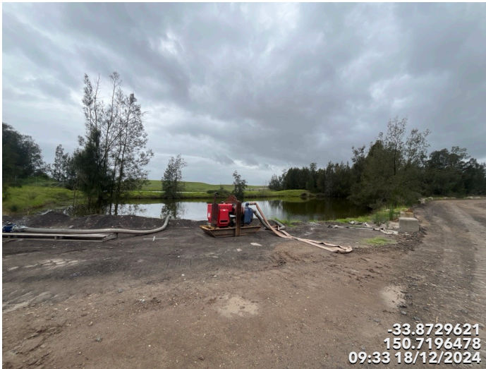
Photo 1 Sediment Basin Water was used for dust suppression
